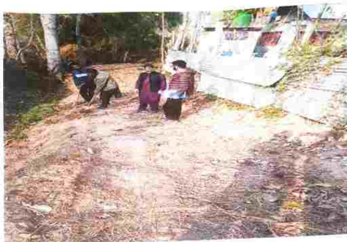
Foundation of Road from Main Road to H/o Farooq Ah Ganaie
