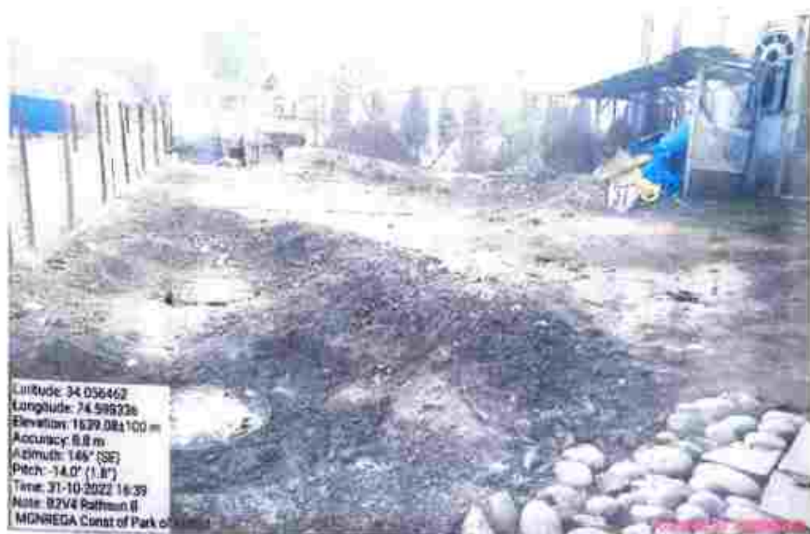
Work under MGNREGA D/D of Park for Masjid Sharief
