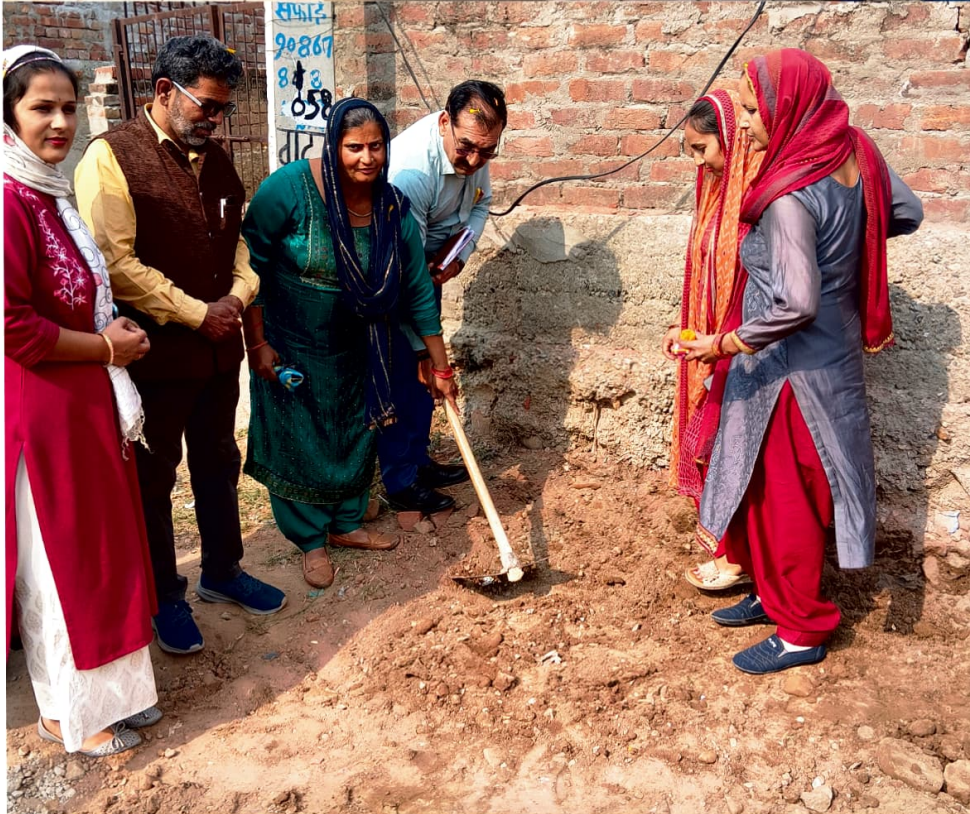
Inauguration & Laying of Foundation Stone of new works By the visiting Officer Sh. Yash Paul Sharma
